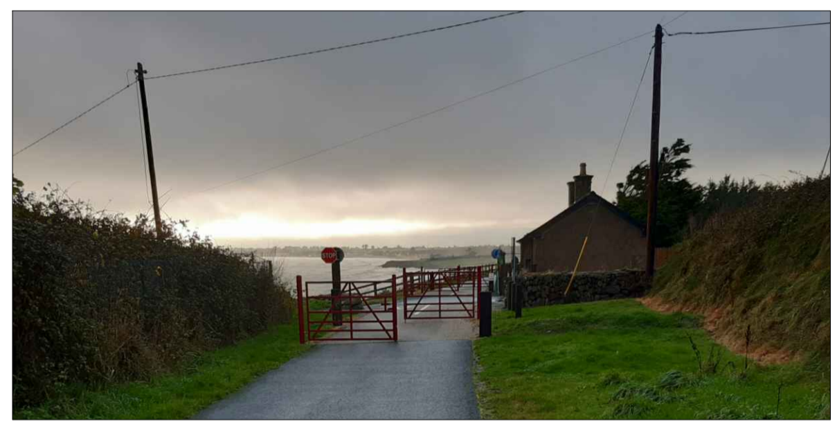
Chicane railings in advance of interactions with public roads
